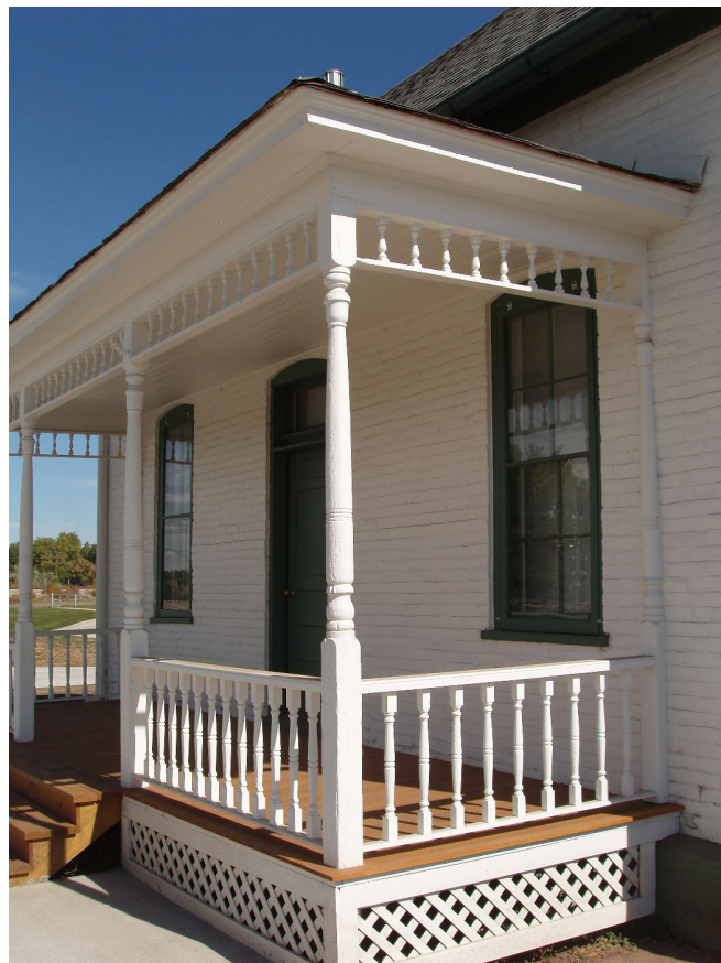
Photo 2 Southeast side of porch, camera facing northwest*
