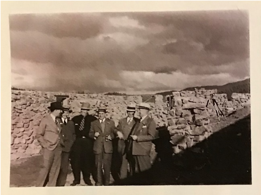
Photo HP02. House construction—foundation wall, estimated between 1940–1942, view to southwest (Gould Family Photo Collection, courtesy of Nancy Kempf).
