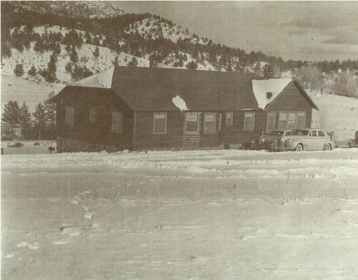
Photo HP08. West and south sides of house, probably 1942, with fishing pond to north in background, camera facing northeast (Gould Family Photo Collection, courtesy of Nancy Kempf).
