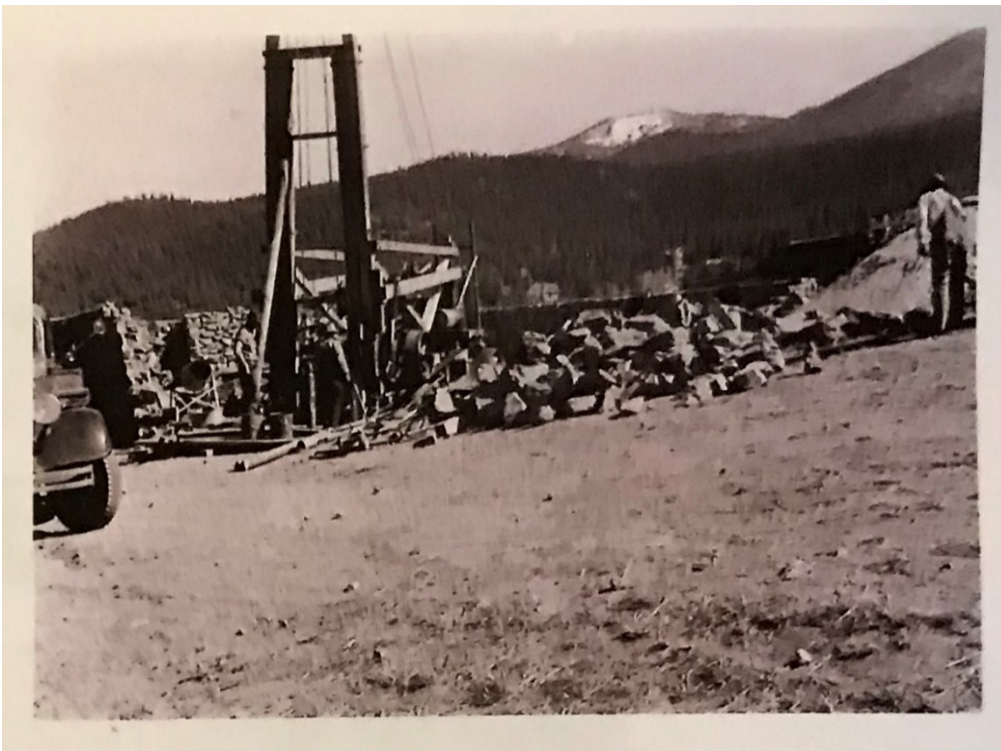
Photo HP03. House construction—foundation wall, (well drilling?) between 1940–1942, view towards Shawnee? (Gould Family Photo Collection, courtesy of Nancy Kempf).
