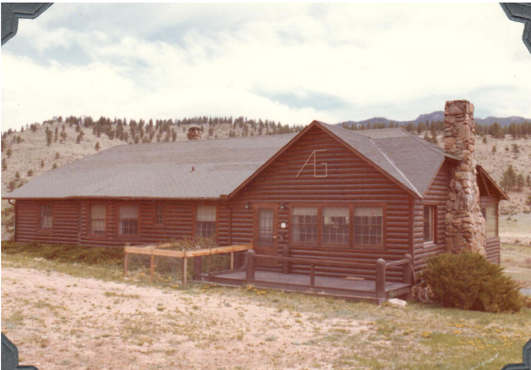
Photo HP13. South and east side of house, camera facing north (USFS Photo, Dargan 1979).
