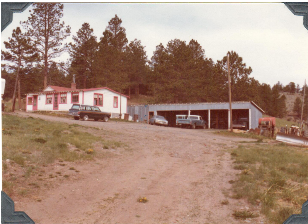
Photo HP23. Caretaker's house and maintenance/machine shed, camera facing to southwest. Shed is extant, caretaker's house was removed in the 1980s (USFS Photo, Dargan 1979:9).
