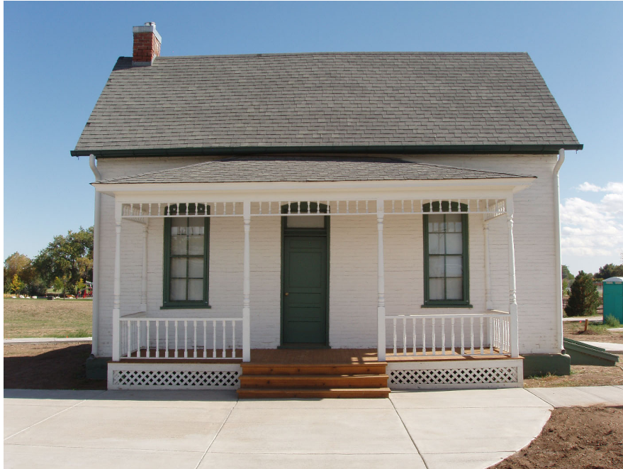
Photo 1 Southwest (main) Façade, camera facing northeast
