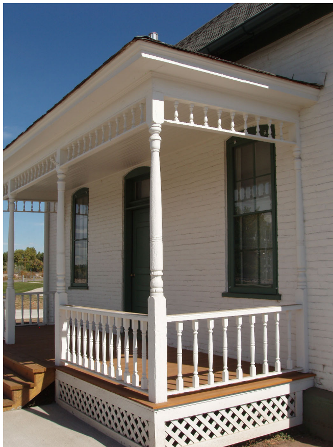
Photo 2 Southeast side of porch, camera facing northwest*
